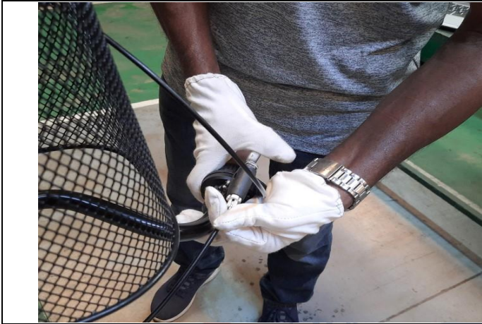
Cable Pinch and bolts Check
