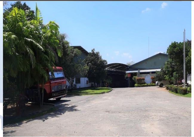
Factory Front View
