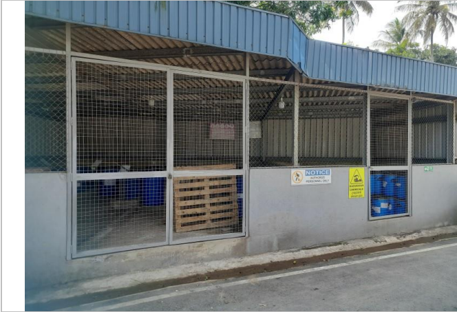
Chemical Storage Area
