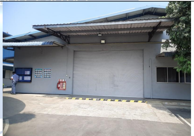
Wearhouse Front View - Lording area
