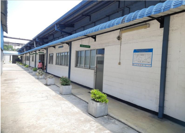
Factory Building view
