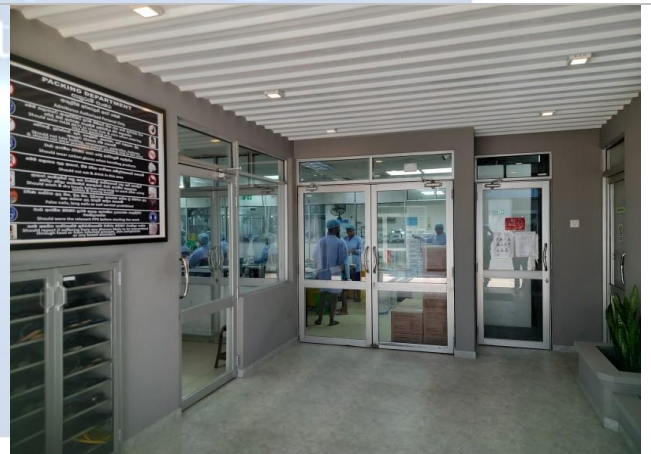
Packing Department Front View
